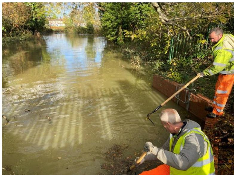
**Figure 3-5 Water level at the trash screen while being cleared by Redbridge contractors. Source: EA**
