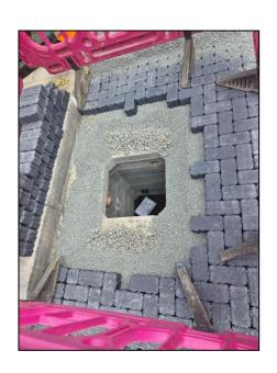
Since its installation in mid-2024, Seven Kings High Road has not experienced the flooding that previously affected the area. The Hydrorock system has performed as expected, preventing flooding even during heavy rains. As a result, Seven Kings High Road businesses have not experienced the disruptions that previously affected the area, which often made it inaccessible during storms. The system also helps reduce pressure on the Thames Water sewer system, benefiting nearby areas as well.
