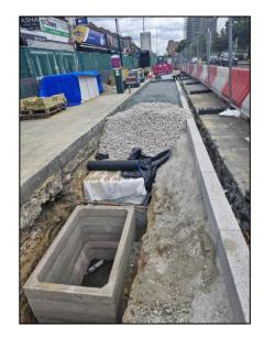
One major advantage of the Hydrorock system is its ability to mitigate flooding without affecting road use. Installed beneath the surface, the system does not reduce parking capacity, a critical factor in busy urban and commercial areas like Seven Kings High Road. Additionally, by holding water and releasing it gradually, the system eases the burden on local drainage infrastructure and reduces the risk of sewer overflows.
