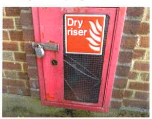
**9.2.4** Compliance certificates were not available to demonstrate that the dry rising main inspections have been completed. Ensure that these are tested in accordance with BS 9990:2006.
