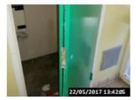
There appeared to be damage to the door. If the integrity of the door is compromised, this could allow the passage of smoke and fire into adjacent areas, which could compromise the means of escape. The missing door lock could also encourage the unauthorised use of this cupboard for storage purposes.
